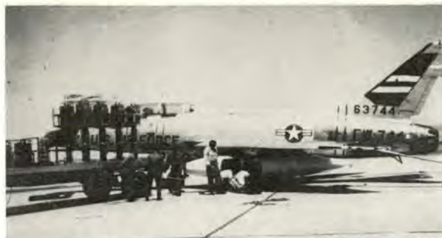
Ground check of lightning data collection equipment on the F-100F.
